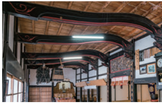
Graceful curved beams
