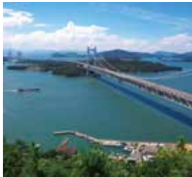
Seto Ohashi Bridge
