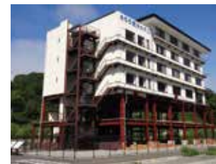
Post-tsunami remains of the Taro Kanko Hotel
