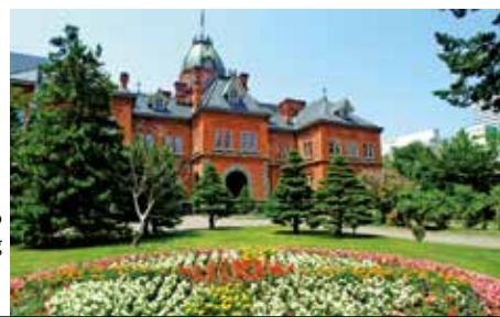
The Former Hokkaido Government Office Building
