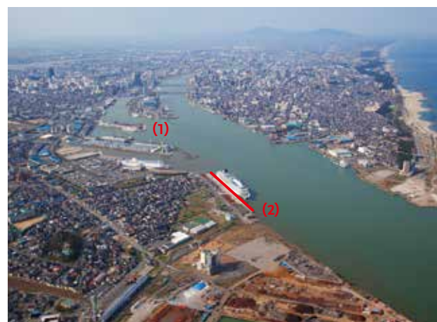
Niigata West Port District
