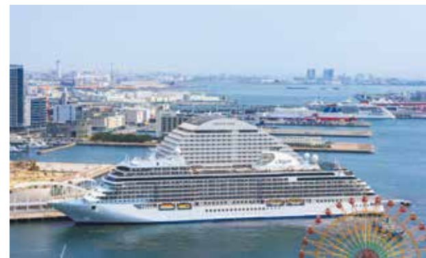
Naka Pier Cruise Terminal
