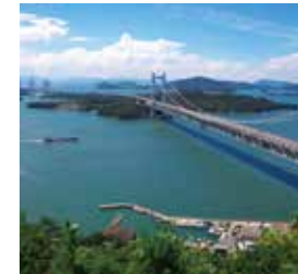
Seto Ohashi Bridge
